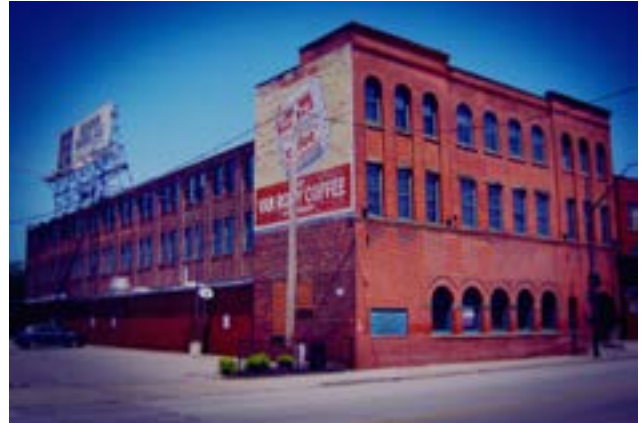
SPACES @ the Van Rooy Coffee Building
